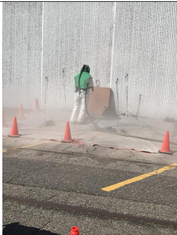
View of: 02-During blasting operation #1
